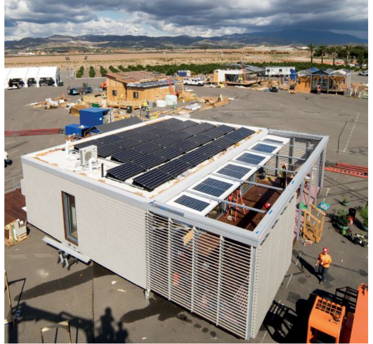
After shipping the house across the country, it was reassembled at the Solar Decathlon site in Irvine, Calif. Photo: Juan Paolo Alicante
