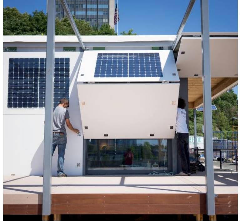
Storm shutters act as protection against storms when down and provide shading and support solar collectors when raised. Photo: Juan Paolo Alicante
