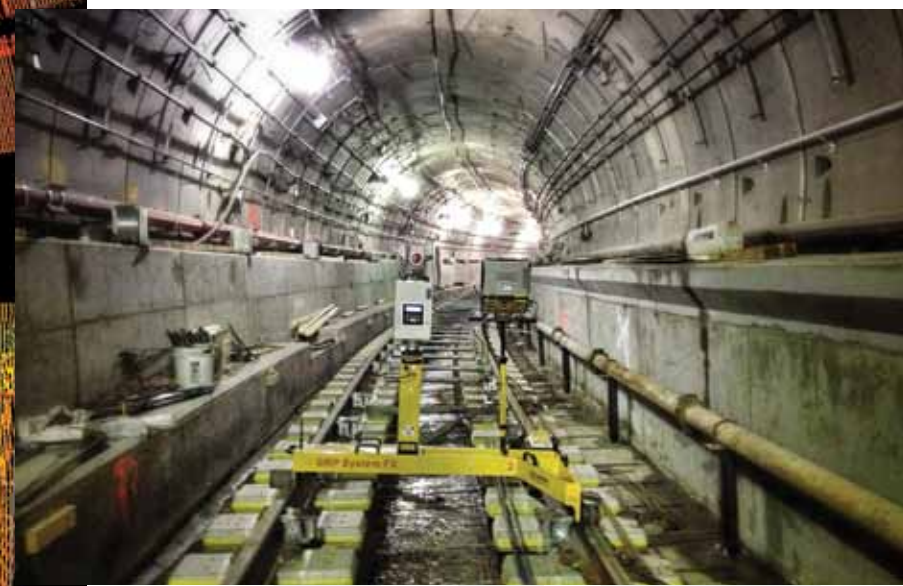
Opposite: Three-dimensional Autodesk AutoCAD drawing exchange format files of tunnel wall cross-sections with Metro Transit Authority car-body data overlaid onto laser scan data for the No. 7 subway extension project in New York City. Left: The Amberg GRP 5000 trolley system takes track as-built scans prior to the pouring of concrete on the No. 7 rail extension project in New York City. Images courtesy of Maser Consulting
